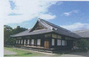
Sei-cho ("Sei" literally means right and formal, and "cho" does an office.) is a hall where large-scale examinations and ceremonies were held in the presence of the lord, while Shizen-do ("Shizen" literally means to practice virtue, and "do" does a hall.) is a facility with rooms for the lord to take some rest and places for the successive lords and their sons including Yoshinobu Tokugawa to devote themselves to their studies.
